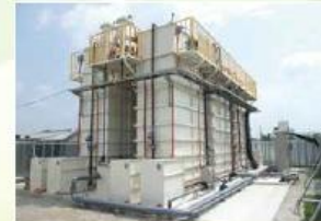
Energy-saving membrane bioreactor pilot test plant
